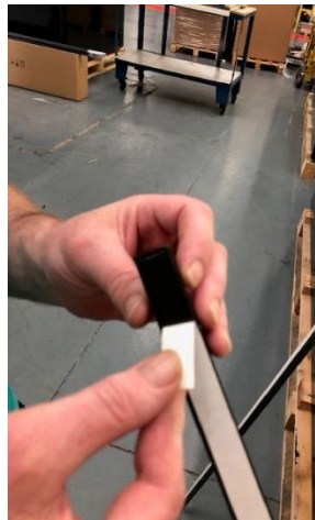
Remove backing from double sided sponge tape
